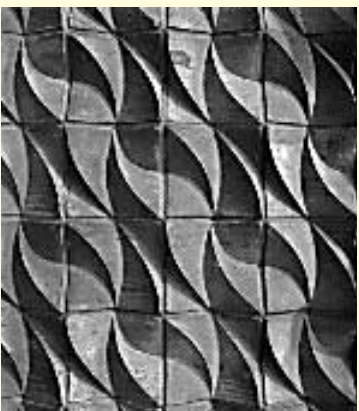
2b Formstein Beton Leipziger Strabe 46 Mitte
